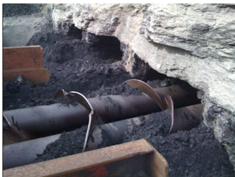
Auger drilling at Mill Creek
